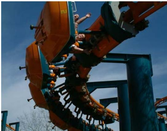
In the spring of 1984, AstroWorld took a chance with Arrow to design and build a suspended roller coaster. The only previous modern attempt to build such a coaster had ended in failure when “*The Bat*” at Kings Island was removed due to structural problems. With these problems solved, mostly due to added banking of the turns, AstroWorld commissioned Arrow to build *XLR-8*. *XLR-8* would be the last brand new coaster for AstroWorld until 1999 when *Serial Thriller* was installed.
