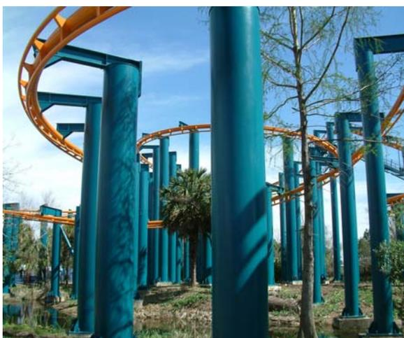
*XLR-8* was 3000 feet long, with a maximum height of 81 feet. Containing two lifts, the ride had a maximum speed of 35 mph. This coaster was built as a family ride and proof that the concept could
